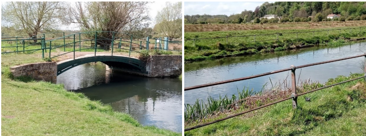
Figure 40 - Estate railings adjacent to New River bridge (left) and along the river (right)
