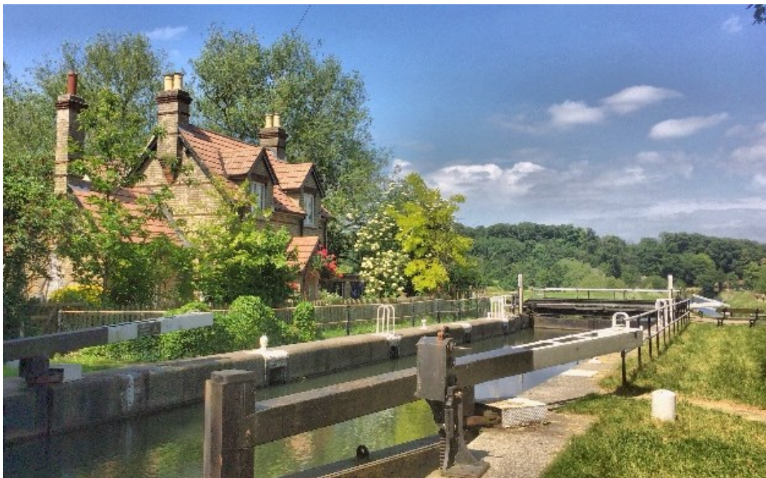
Figure 38 – The Lock House
